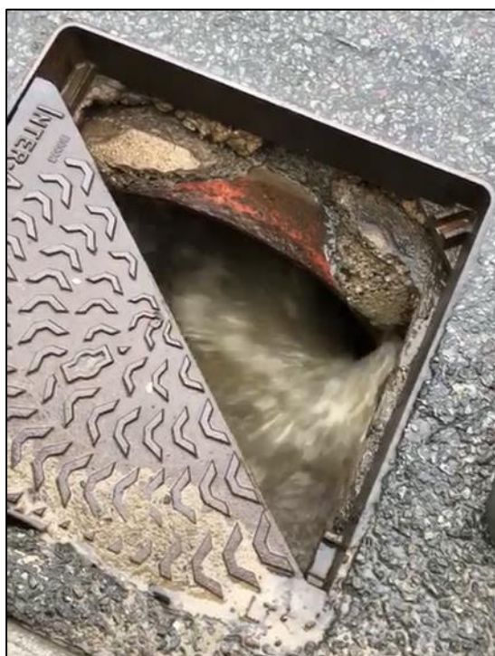
Figure 10: Photo of 'Manhole 1' surcharging during Storm Jorge (captured by RCT's Flood Risk Management team on 28 th February 2020)
