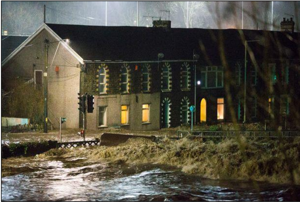
Figure 5: Photo of the rapid onset of flooding from the River Taf at Cardiff Road during Storm Dennis (Image: Wales Online)
